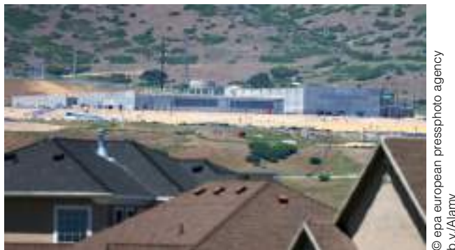
FIGURE 2.17 The NSA data center in Bluffdale, UT.
